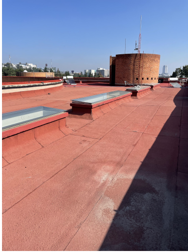
Figure 1: Waterproofed roof at UIA
